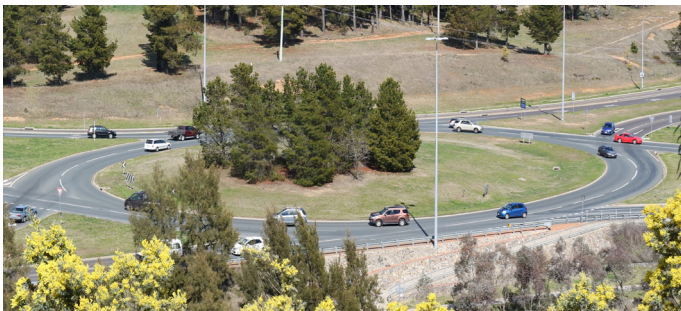
Overlooking the Barton Highway/ Gundaroo Drive/William Slim Drive roundabout
