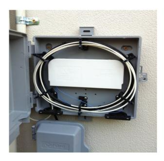
The conduit takes the fibre up to the ceiling space, & is snug behind a downpipe so is minimally ugly, less so after a lick of house paint. Inside this cable is the actual fibre-optic "cable" that carries this incredibly fast bandwidth. What does this look like?
